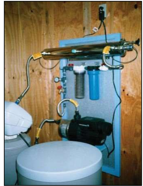
UV Light (top horizontal cylinder) Texas Rainwater Manual
