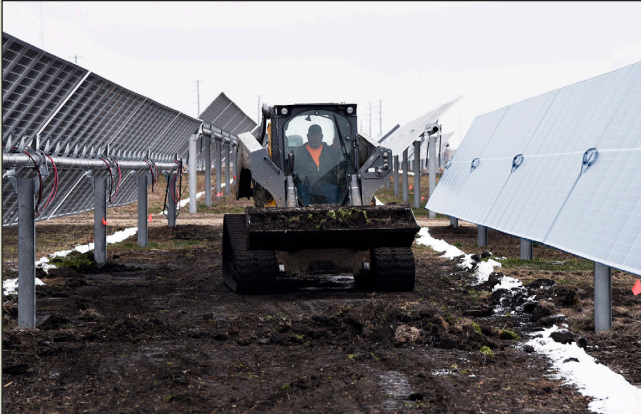
Installation of the Solar Farm 2.0 array included 31,122 panels that can track the path of the sun. Each panel on each row is on a north-south single axis self-powered tracker that allows for more efficient collection of solar power.
