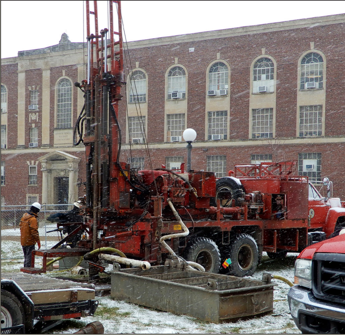
Core samples taken at the geothermal energy drilling site at the Campus Instructional Facility (CIF). Geothermal energy will help the CIF use less energy to heat and cool the building, reducing energy consumption, carbon footprint, and expenses in the long run.
