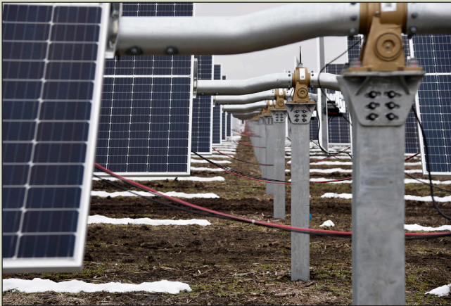
Installation of the Solar Farm 2.0 array included 31,122 panels that can track the path of the sun. Each panel on each row is on a north-south single axis self-powered tracker that allows for more efficient collection of solar power.
