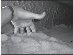
Debris in the air ducts, like the one pictured above from Turner Hall, severely reduce building systems' ability to run at peak efficiency. Retrocommissioning identifies problems like these to save energy on campus.
