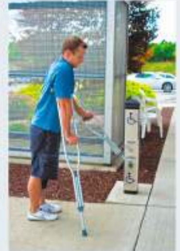
Push buttons need to be within hand reach of wheelchair users and also near the ground level so that it can be operated by users with disabilities
