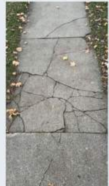
Cracks- more than 4 feet of accessible sidewalk (Count: 350)
