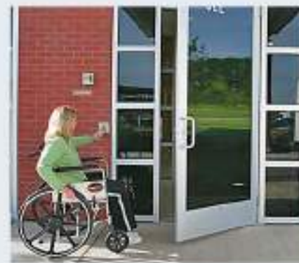
Push buttons need to be within hand reach of wheelchair users and also near the ground level so that it can be operated by users with disabilities
