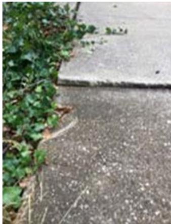
Figure 10 - Vertical Fault
