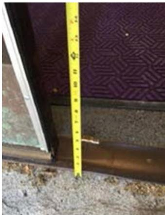
Figure 15 – High Threshold
